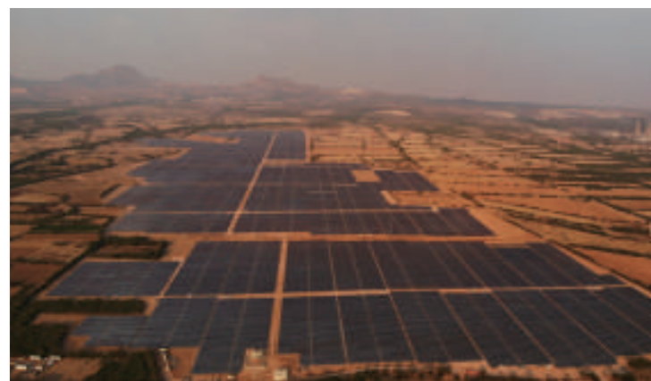
Aguascalientes, Mexico 133MW ground-mounted power station project
