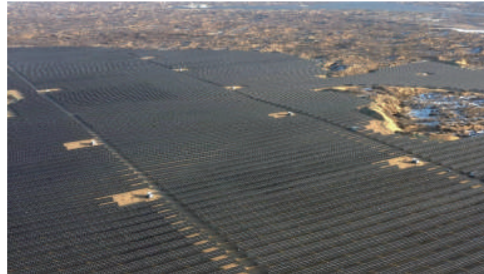
Yulin, Shaanxi Province 100MW Vertex ground-mounted power station project
