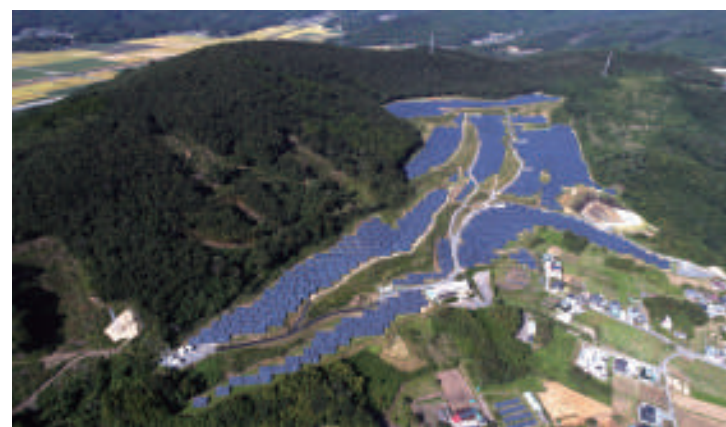
Ishinomaki, Miyagi Prefecture, Japan 14MW ground-mounted power station project
