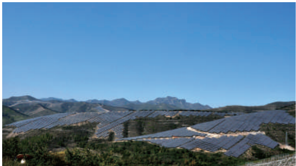
Yangquan, Shanxi 50MW pioneer project
