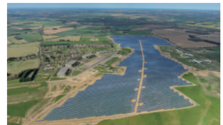
Norfolk, Britain 50MW ground-mounted power station project
