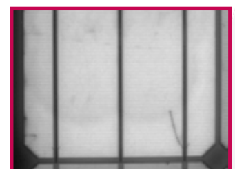
Micro crack between bus bars
