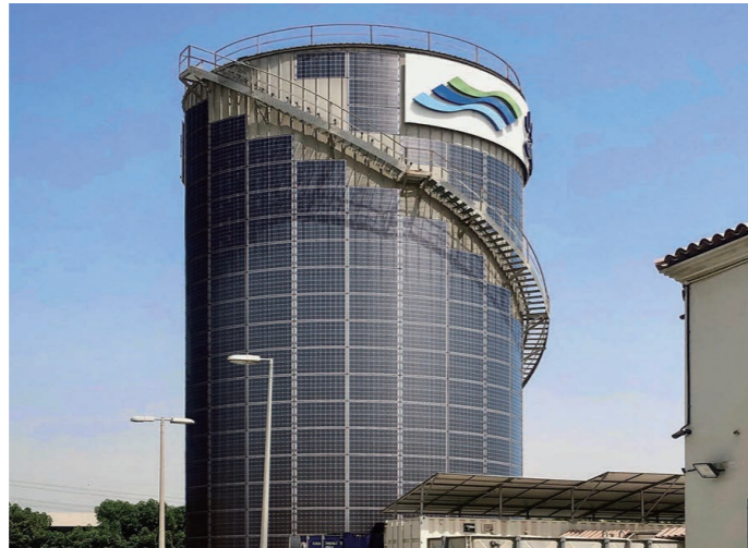
Solar Façade UAE | 50kW
