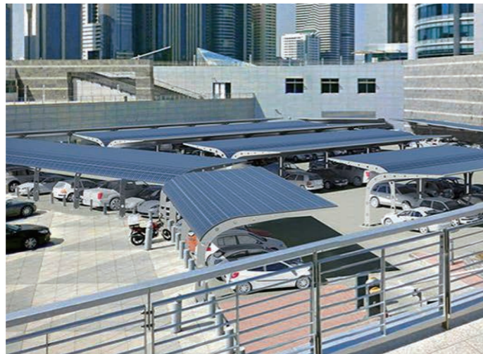
Curved Carport UAE | 273kW
